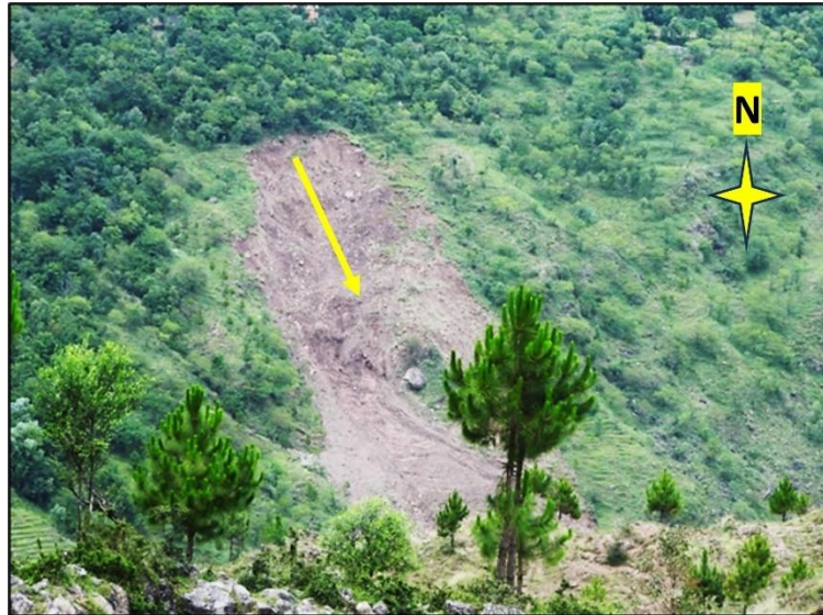
Figure 9: Nammal-IV landslide, just opposite to the Nammal-II landslide.
